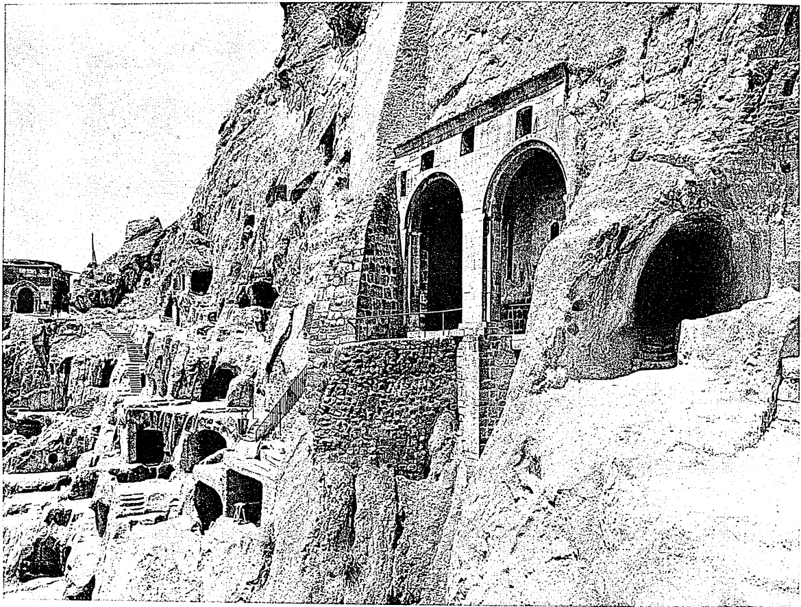
Fig. 54. Vardzia. Church of the Dormition. Exterior from southeast (1184–86).
