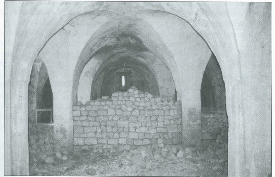
Fig. 15. New constructed wall within the old Armenian church of Yoğunluk
