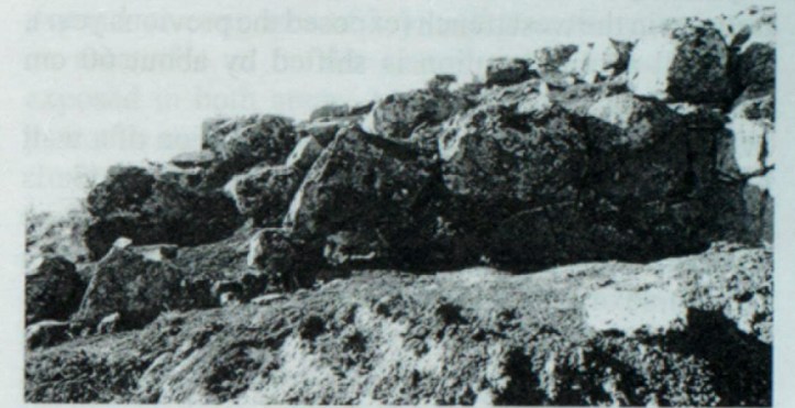
Fig. 12: North facade of stonewall M13.
