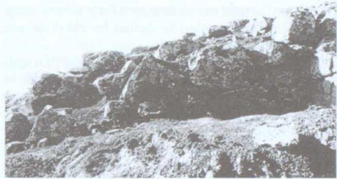
Fig. 12: North facade of stonewall M13.
