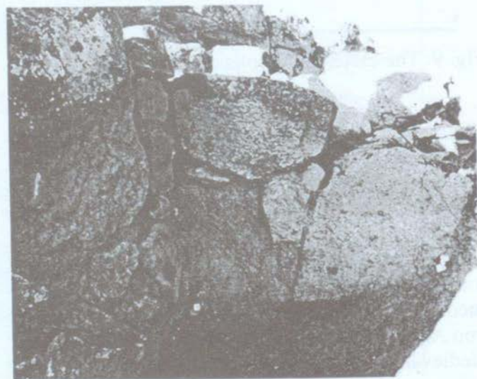
Fig. 11: Connection point between stonewall M13 and the fortress wall of the lower town (right).
